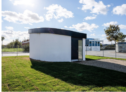
FIRST 3D PRINTED BUILDING IN EUROPE COBOD - Denmark 2017
