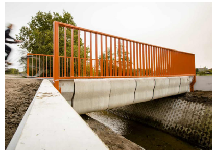
FIRST 3D PRINTED BRIDGE TU Eindhoven - Netherland
