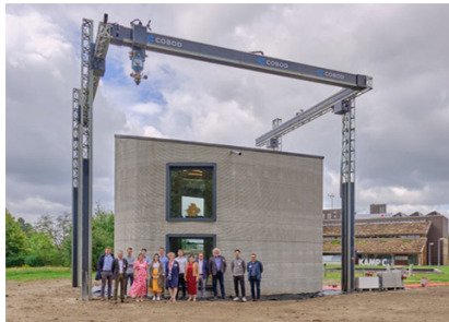
FIRST PRINTED MULTIPLE STOREYS BUILDING COBOD - Denmark
