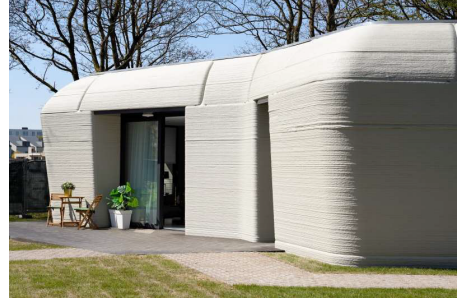
FIRST COMMERCIAL HOUSING PROJECT TU Eindhoven 2021
