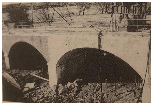
Figura 3.16 Rotherham road railway bridge : prospetto. [46]
