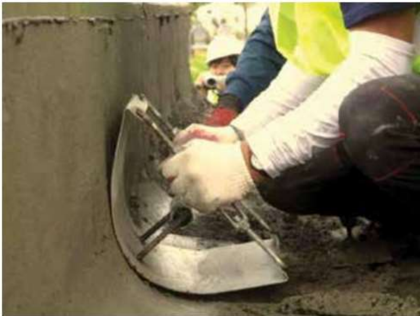
Fig. 5: Finishing radius cove of low wall with a custom-built tool
