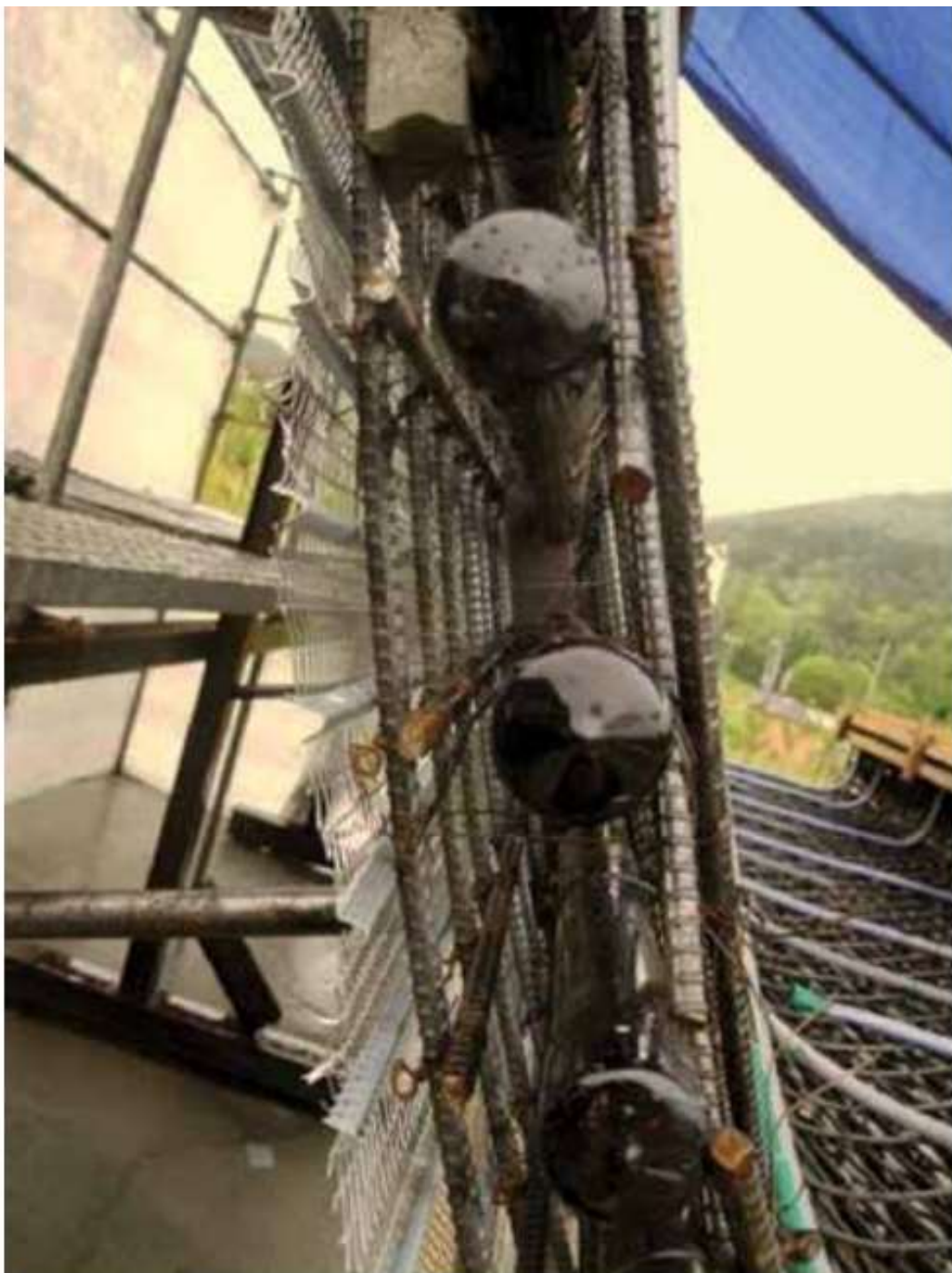
Fig. 2: End view of reinforcing steel, cooling pipes, and Stay Form
