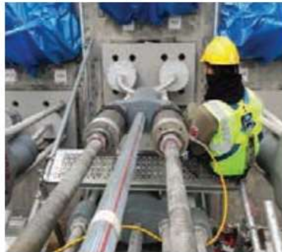
(e) Anchoring at anchor block
