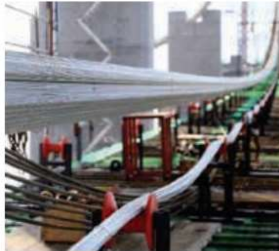
(b) Pulling on catwalk
