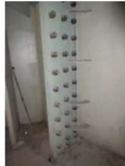
Figure 5: Division of blocks in two or four subpanels and bolted panel connection
